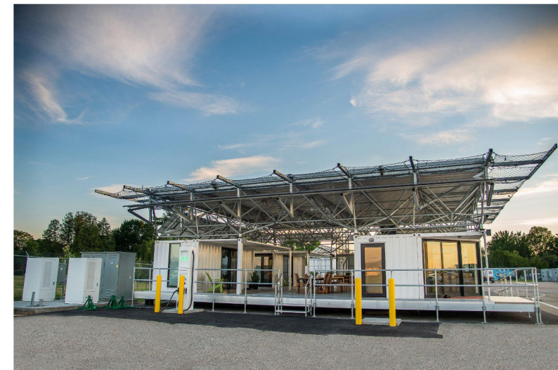
Example eVTOL landing facility with crew accommodations, BETA HQ - Burlington, VT USA
