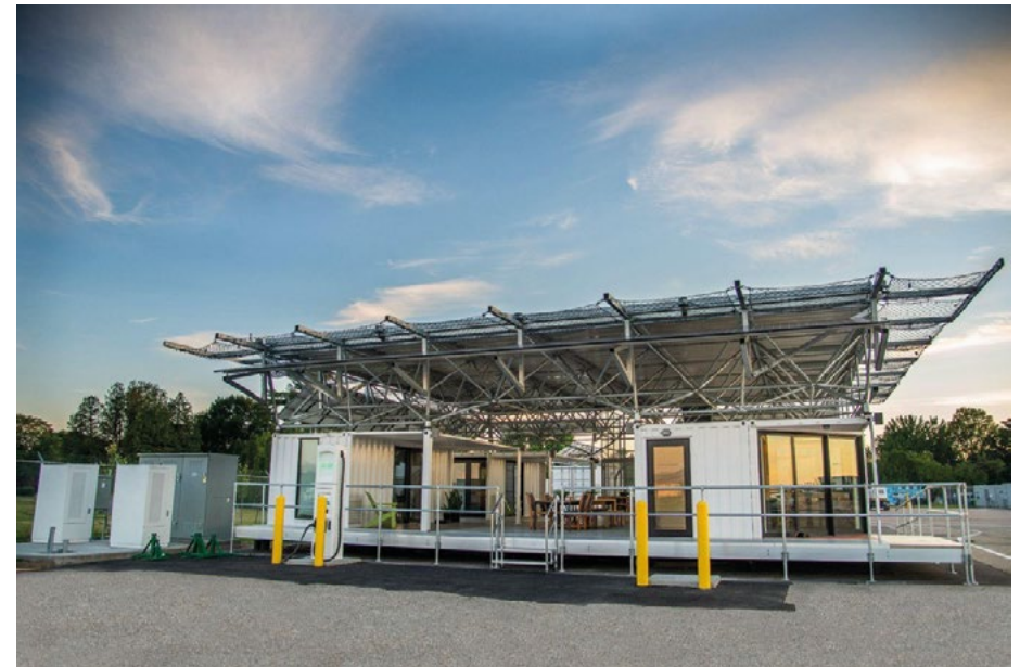
Example eVTOL landing facility with crew accommodations, BETA HQ - Burlington, VT USA
